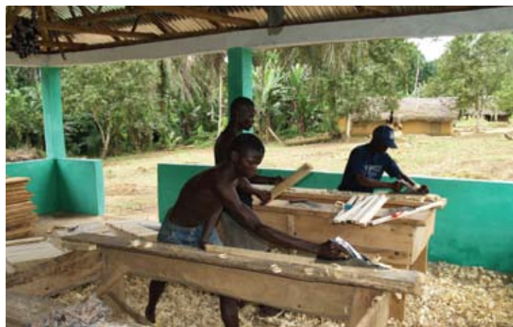
Carpentry workshop, Sierra Leone
