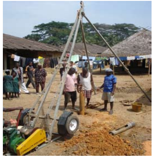
Drilling for Water, Pujehun
